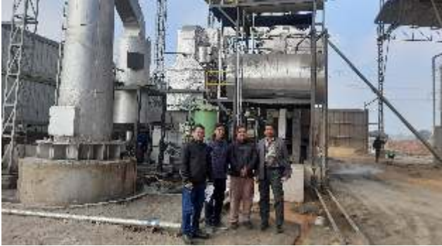
Assessment of Boiler Performance
