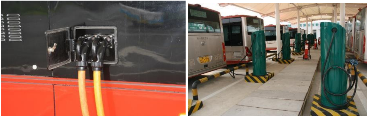
Figure 24: Slow AC Chargers (Type 2) for BEBs
