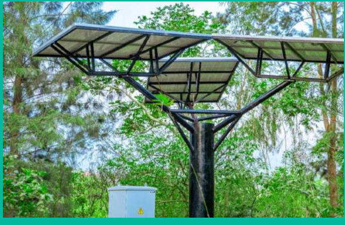
GGGI TEAM RWANDA VISITING THE WETLAND PARK AFTER COMPLETION
