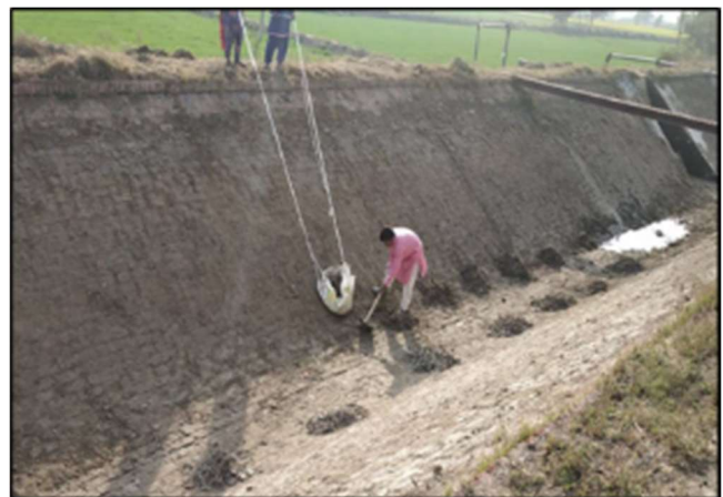
Figure 21: Desilting of canal in Nathushree-Chopta
