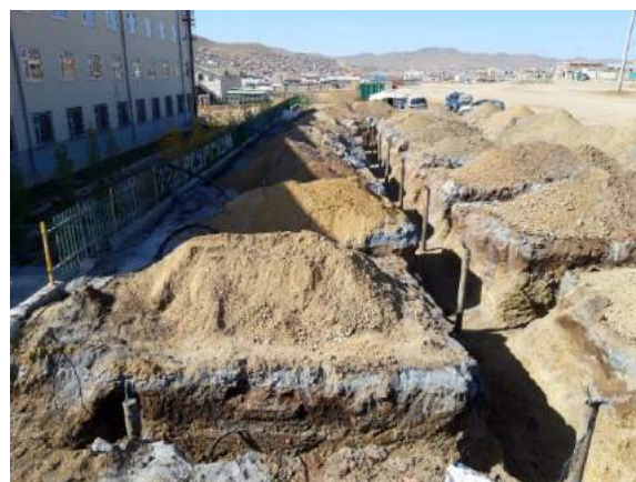
Figure 9 and Figure 10 : Installation of Ground Source Heat Pump of 122nd Public School of Ulaanbaatar city, October 5, 2019. Photo credit to Green Solar Energy LLC
