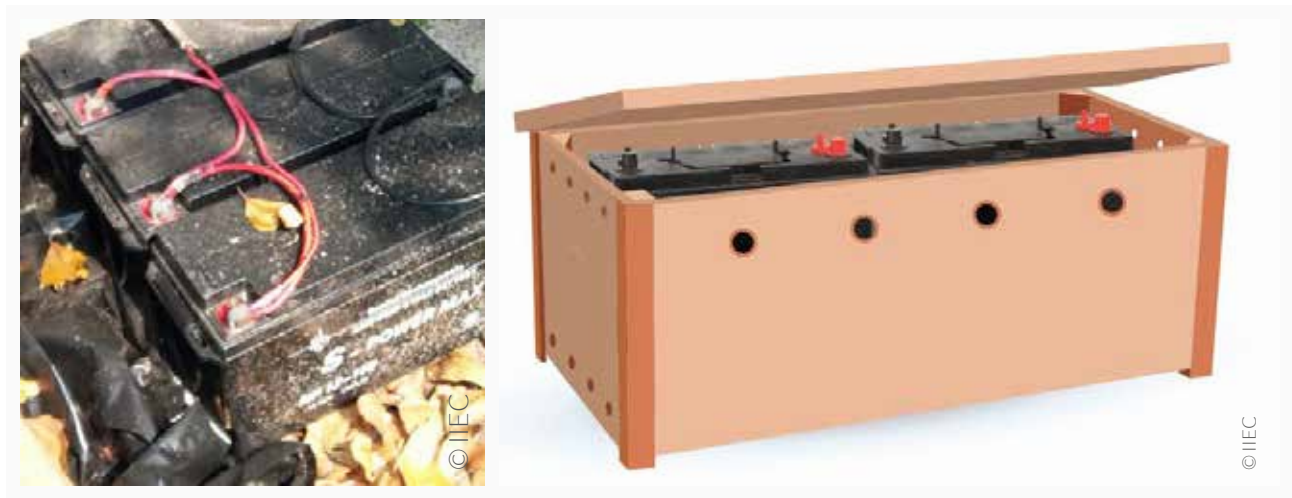
FIGURE 3.2 Outdoor installation of solar batteries (left) and recommended battery box (right)
