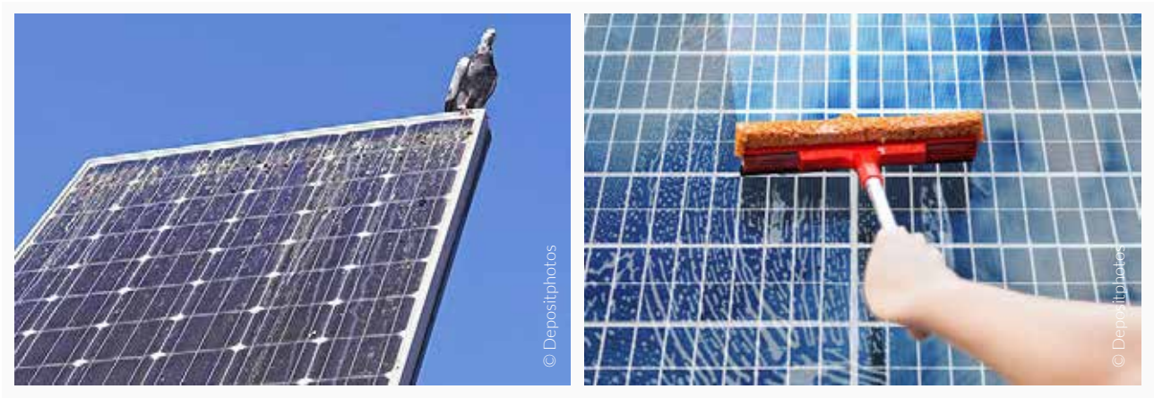
FIGURE 3.1 Dirty solar panel (left) and cleaning of solar panel (right)
