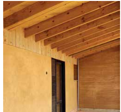
Figure 2: Compressed Stabilized Earth Block (CSEB) wall, rammed earth wall and timber roofing at Rwanda Institute for Conservation Agriculture (RICA) Campus in Bugesera, Rwanda (Representational image of green building)
