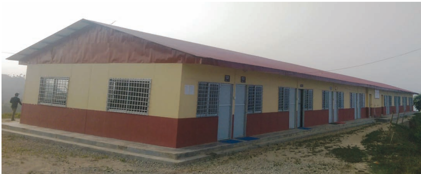
Belkotgadhi Municipality office
